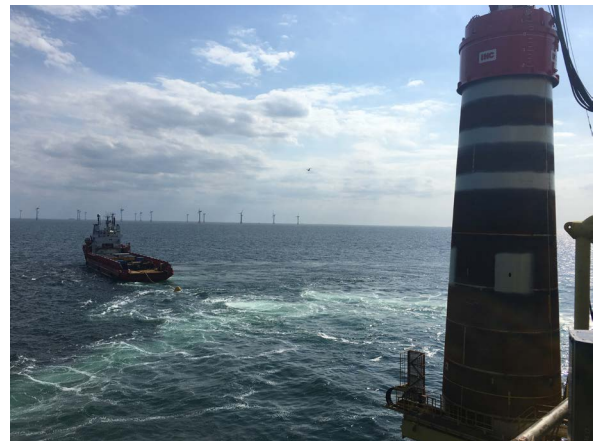
Figure 3. Big Bubble Curtain active during the construction of Rentel.
