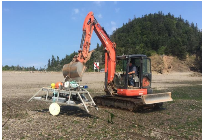
Figure 3: FAST-EMS being put into place for low flow/intertidal testing.
