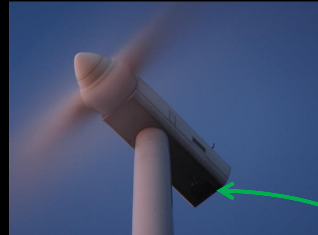
UV illuminators on bottom and top of turbine nacelle
