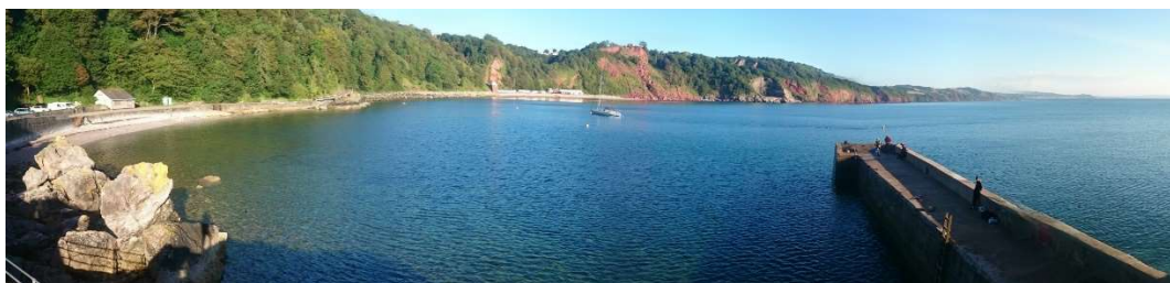
Figure 3.1. Babbacombe beach and breakwater.
