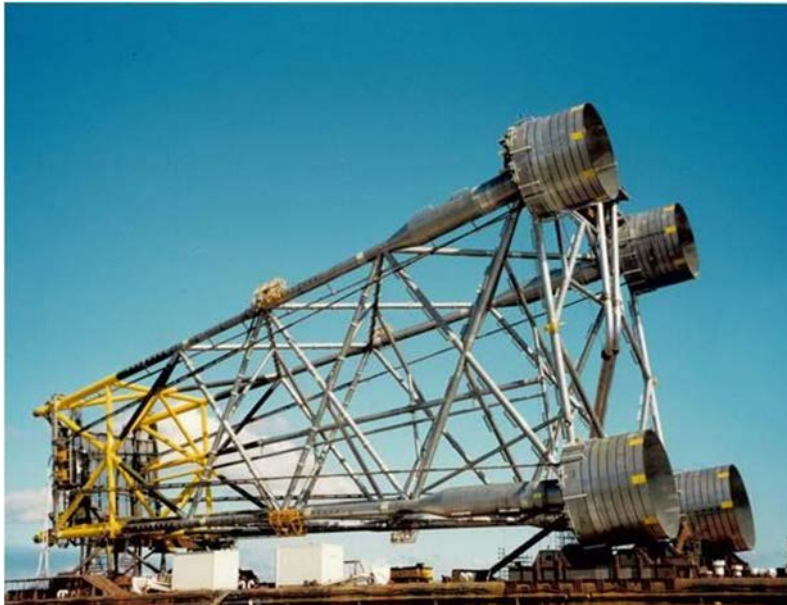
Figure 3.10 Example of a suction bucket multileg foundation
