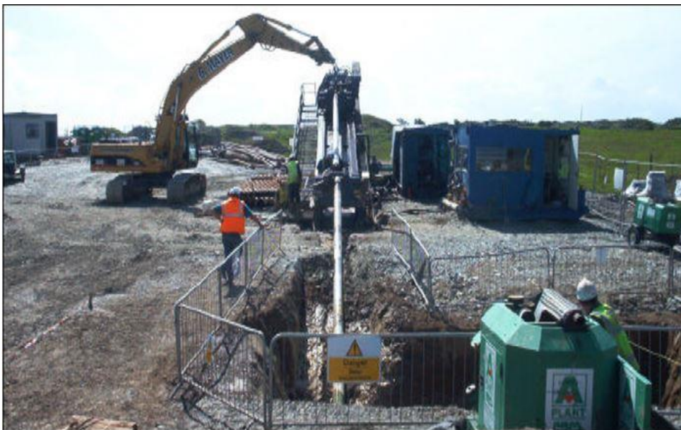
Figure 4.2 Example of typical HDD equipment
