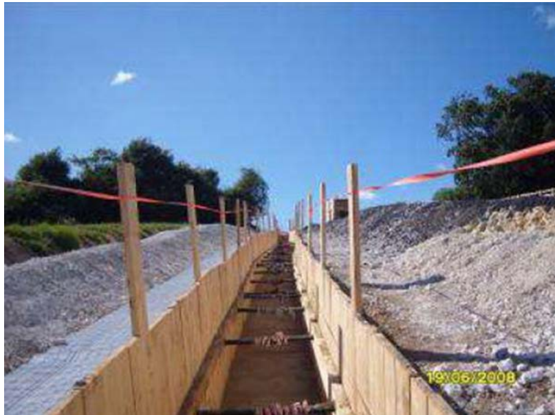
Figure 4.9 Example of close timbered trench
