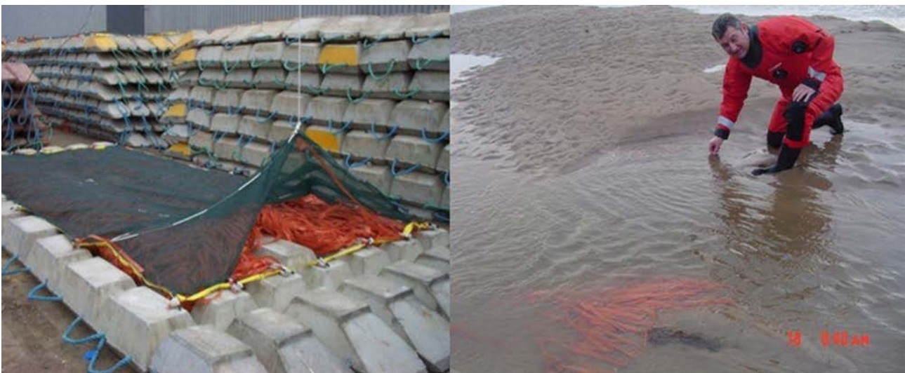
Figure 3.42 Illustrative example of a frond mat, and operational effects
