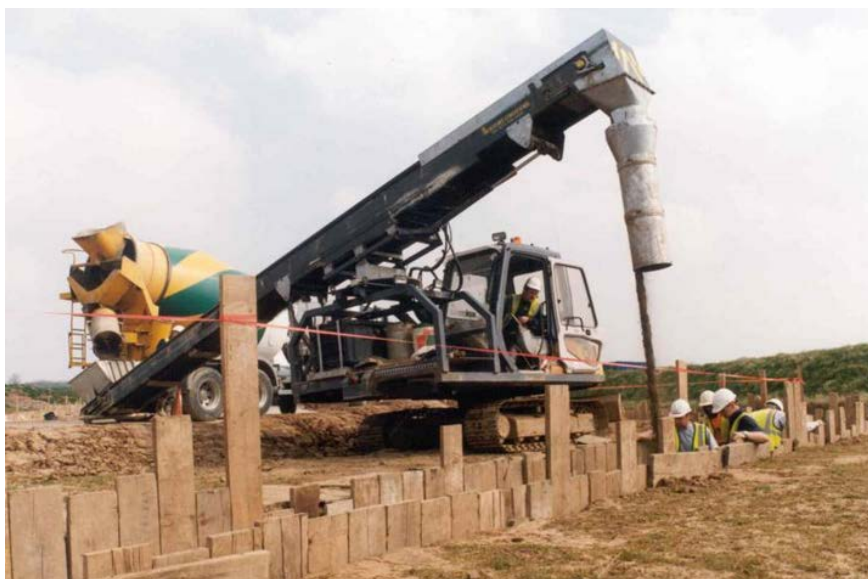
Figure 4.21 Example of a cement bound sand delivery
