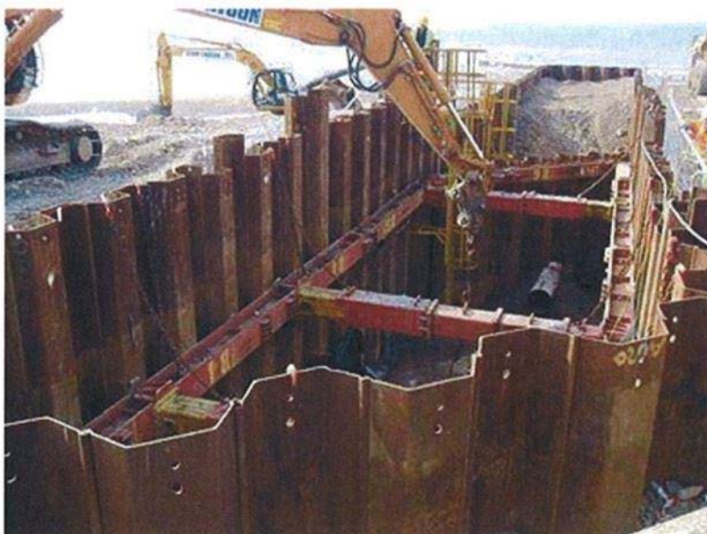
Figure 4.3 Example of a sheet piled cofferdam being installed on a beach
