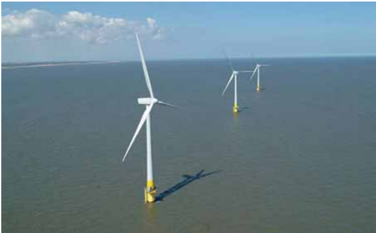
Figure 1.0 Scroby Sands offshore wind farm
