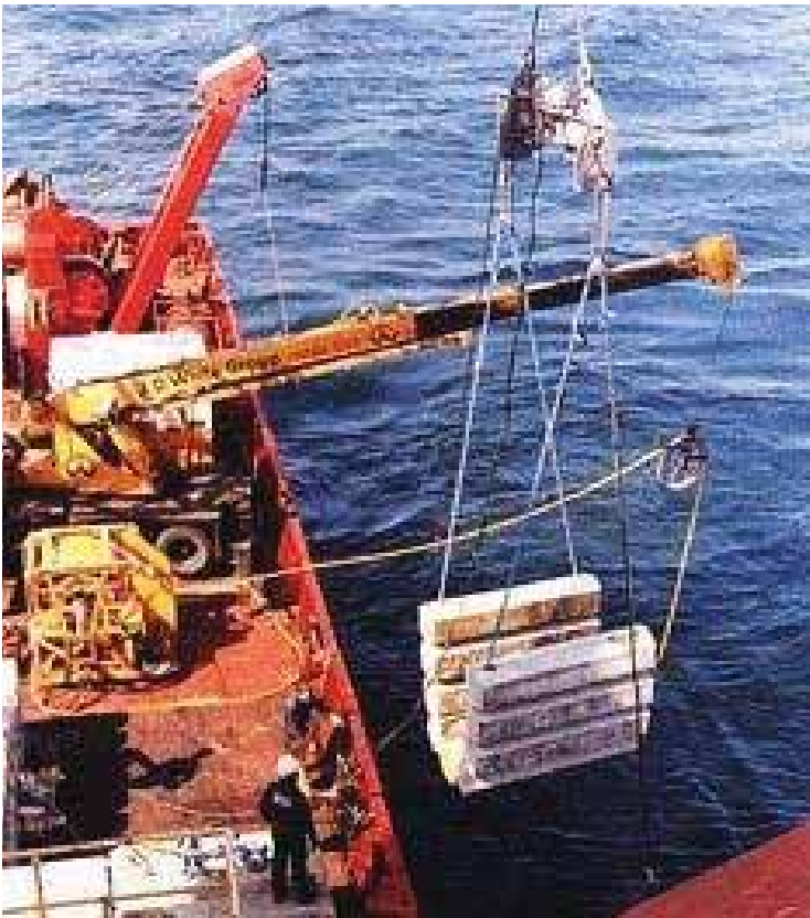
Figure 3.24: Concrete Mattress being deployed by Crane from a Host Vessel
