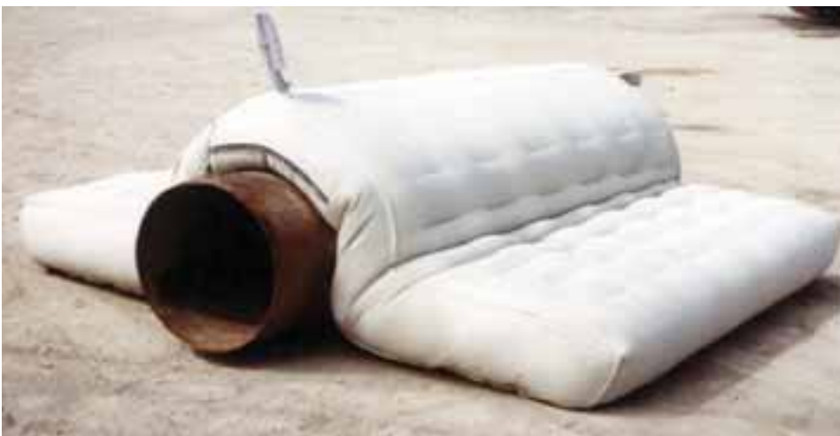
Figure 3.27: Grout Bag over a Pipe Section and Filled with Grout
