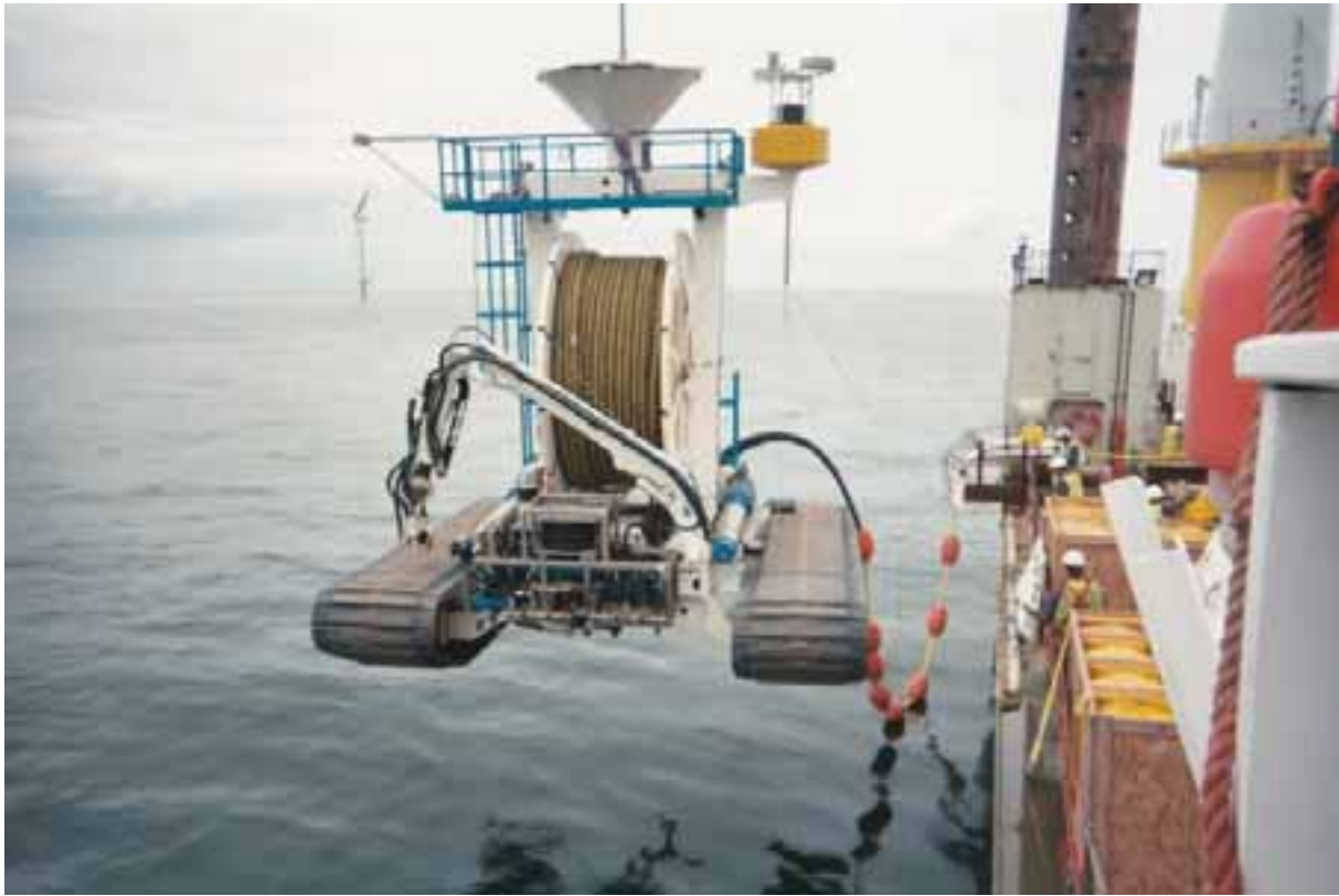
Figure 3.19: LBT1 being deployed at the North Hoyle Offshore Wind Farm Site
