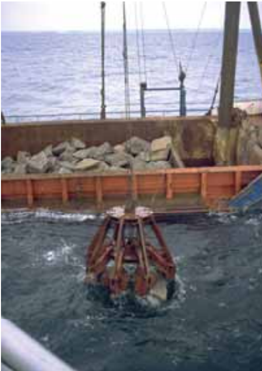
Figure 3.26: Placement of Rock for Scour Protection
