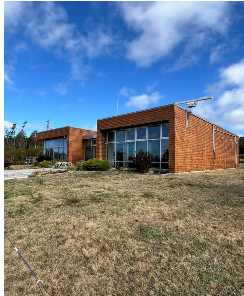
The FORCE Visitor Centre occupies a cleared landscape within a broader transition between upland ridges and valley corridor habitats.
