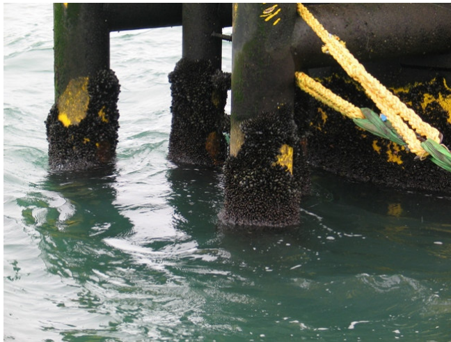
Figure 12. Detail of the fouling near the splash zone of WTG-08.
