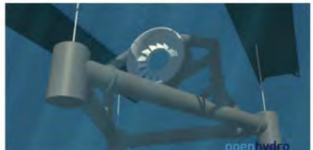
While being held in place by the tug, the turbine and subsea base are lowered by the installation barge.
