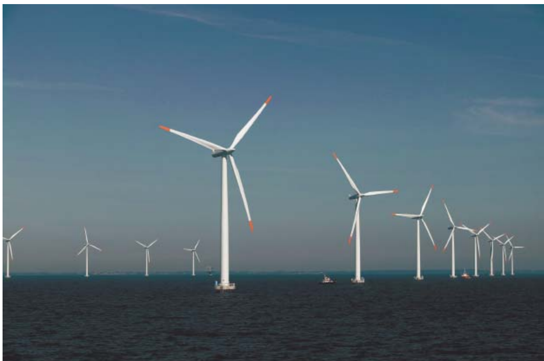
Fig. 1.4: Nysted offshore wind farm (photo: Energi E2).
