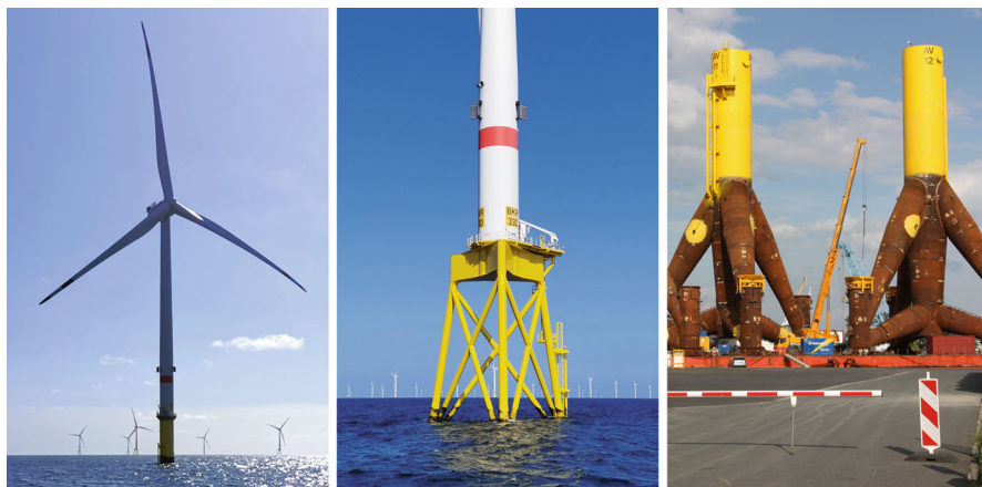
Fig. 1 Monopile, jacket, and tripod turbine foundations (from left to right). (Photos: itap)
