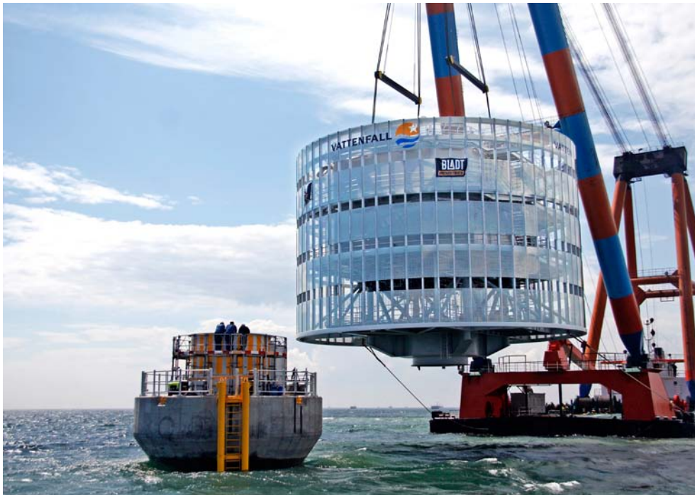
Picture 5. Installation of transformer station at Lillgrund (Photo: Hans Blomberg/Vattenfall).
