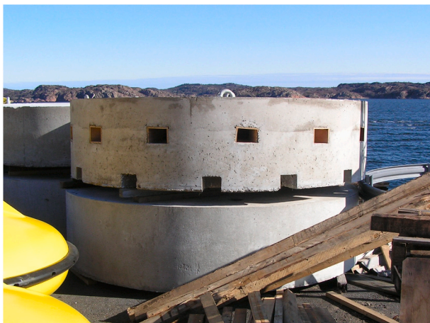
Fig. 2. Foundations surveyed during the study. Upper foundation represents complex version with manufactured holes and lower foundation represents non-complex version.
