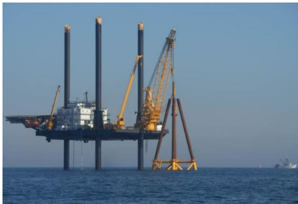
Figure 1-3 Jack-up piling barge with four piles inserted, not driven, and hammer ready
