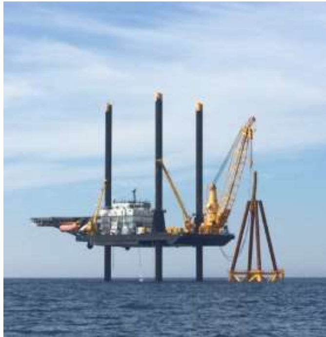
Figure 7. One of the foundations of the Block Island Wind Farm is shown to the right of the Lift Barge Robert.
