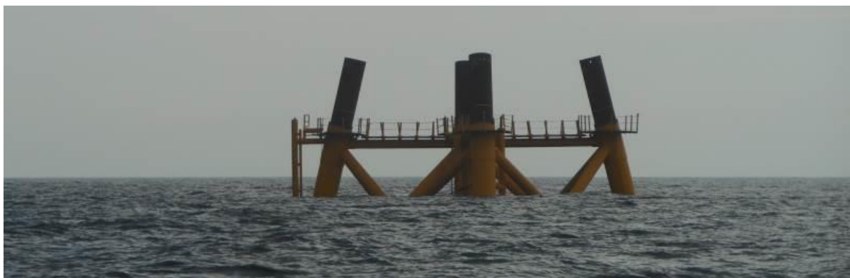
Figure 1-4 Jacket with four driven piles
