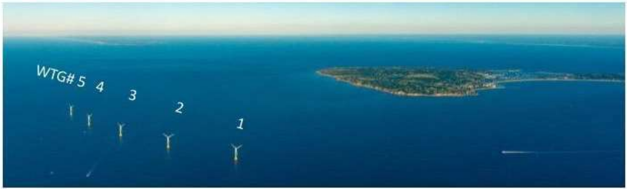
Figure 6. An aerial view of the Block Island Wind Farm and Block Island. The numbers refer to the ID numbers from Table 1.
