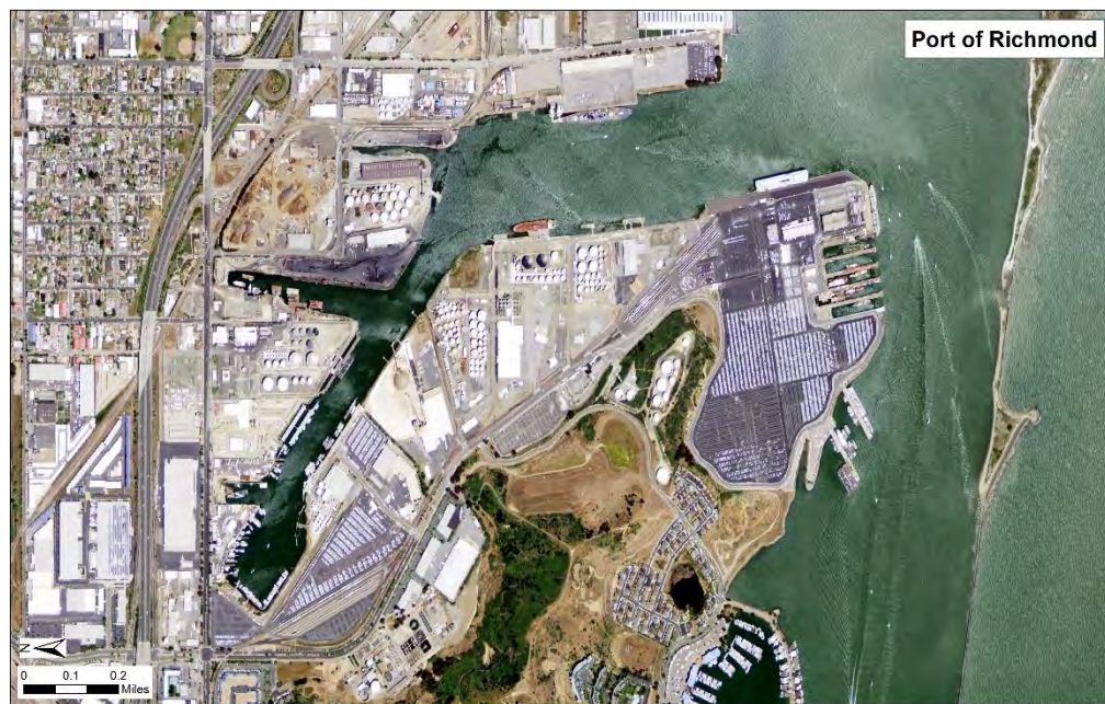
Figure A-6. Port of Richmond.
