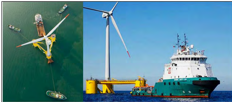
Figure 3-3. Semi-Sub demonstration project installation (WindFloat, 2014)
