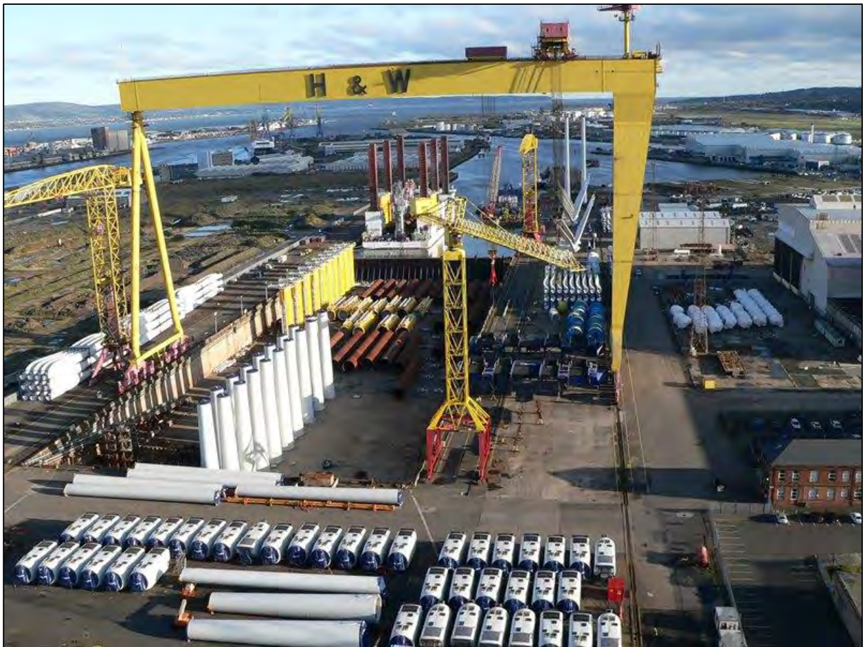
Figure 2-12. Example offshore wind staging area with land-based crane >300 ft. in height (Harland and Wolff 2010)
