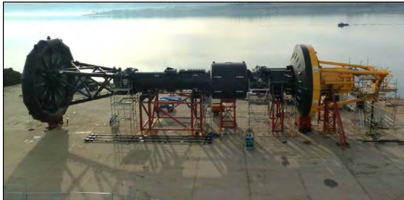
Figure 4-6. Example of staged full-size MHK device using scaffolding (Hug Energy Inc. 2015)
