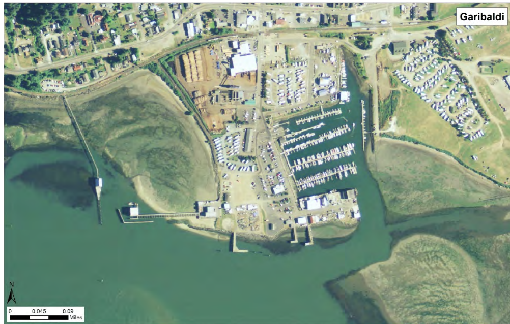
Figure A-16. Port of Garibaldi
