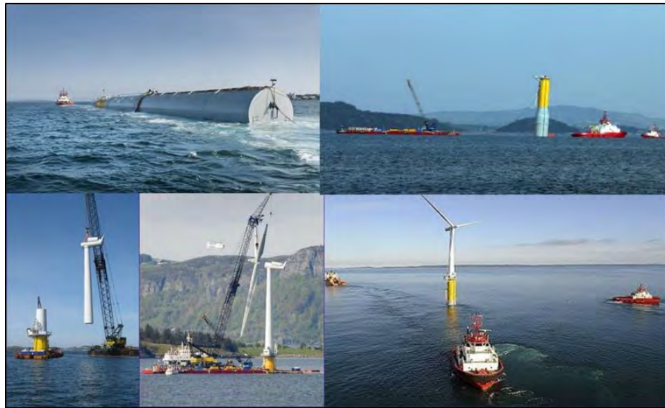
Figure 3-4. Spar demonstration project installation example (Hywind 2015)
