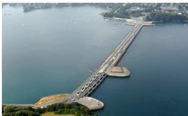
Fig. 1. Example of La Rance Tidal Barrage structure in France ( The Ecologist, 2010 ).
