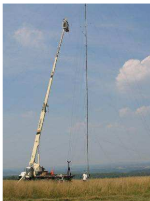
B. Boom truck used to mount pulley system
