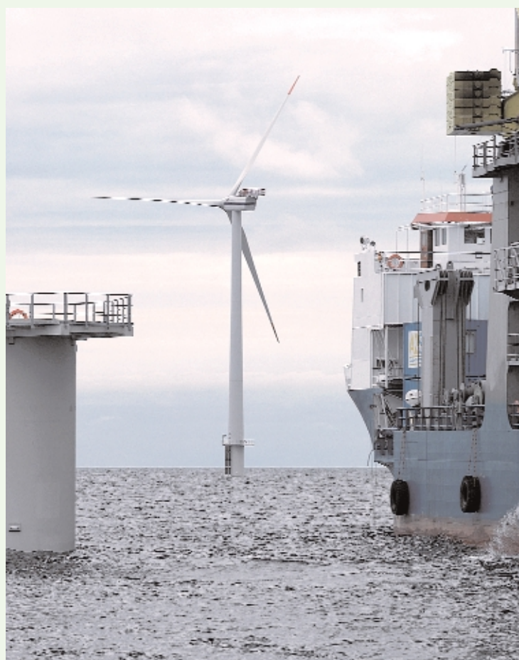
Support vessel at Horns Rev wind farm, Denmark
