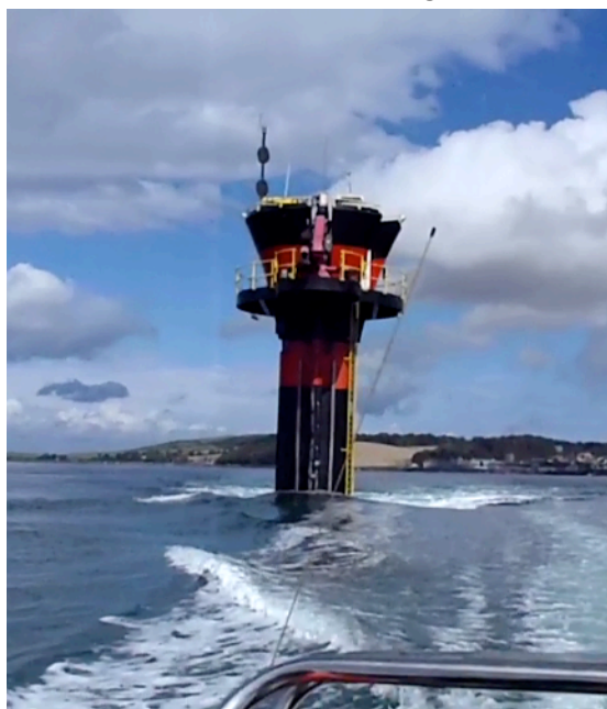
Marine Current Turbines' 1.2 MW device at Strangford Lough in Northern Ireland.
