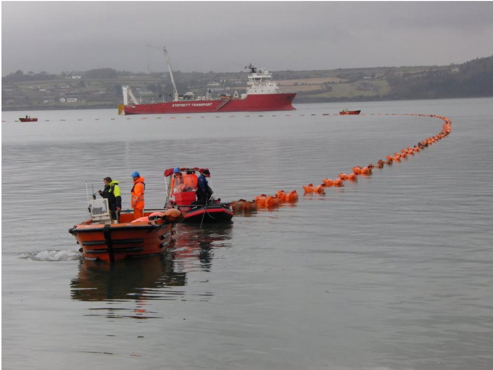
Figure 4-23: Shallow water cable deployment
