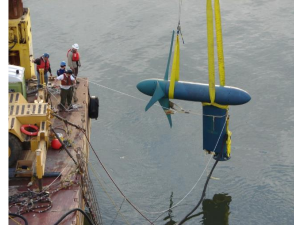
Verdant Axial-Flow Turbine
