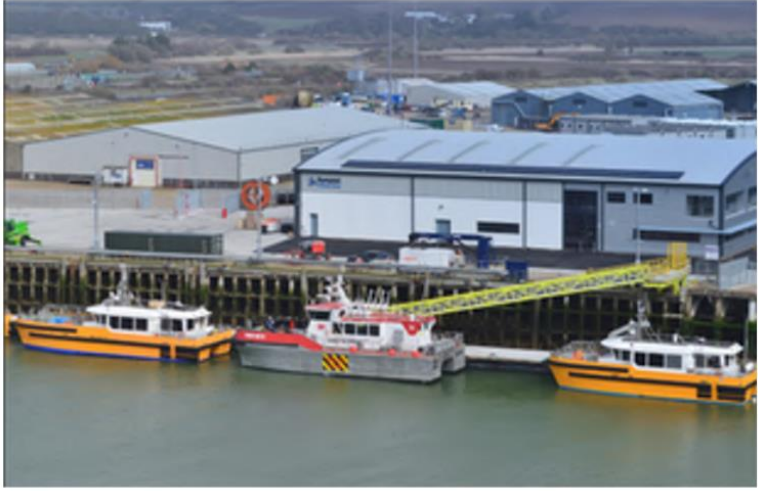
Operations & Maintenance (O&M) Port
