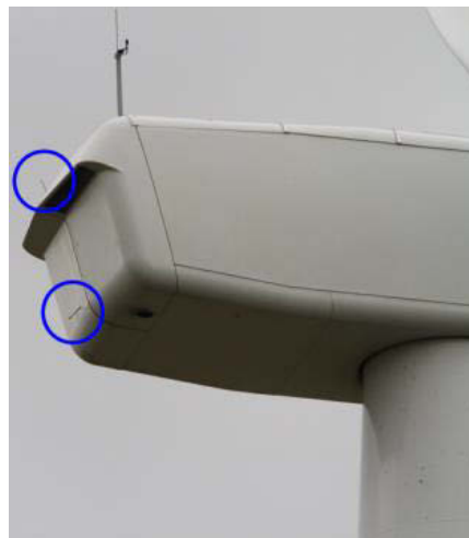
Rear nacelle mounted emitters
