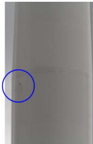
Tower mounted emitters
