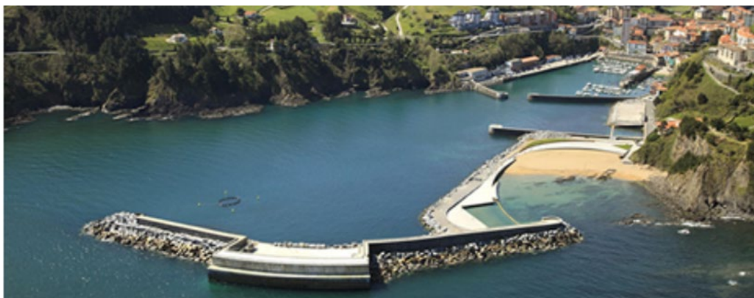
Figure 5.4. The Mutriku Wave Power Plant opened in July 2011 and provides harbor protection while generating electricity by harnessing air compressed by the action of waves, showing a positive benefit of MRE devices. The plan has 16 turbines with a total capacity of 296 kW (Ente Vasco de la Energía, http://www.eve.eus/Proyectos-energeticos/Proyectos/Energia-Marina.aspx?lang=en-GB ).
