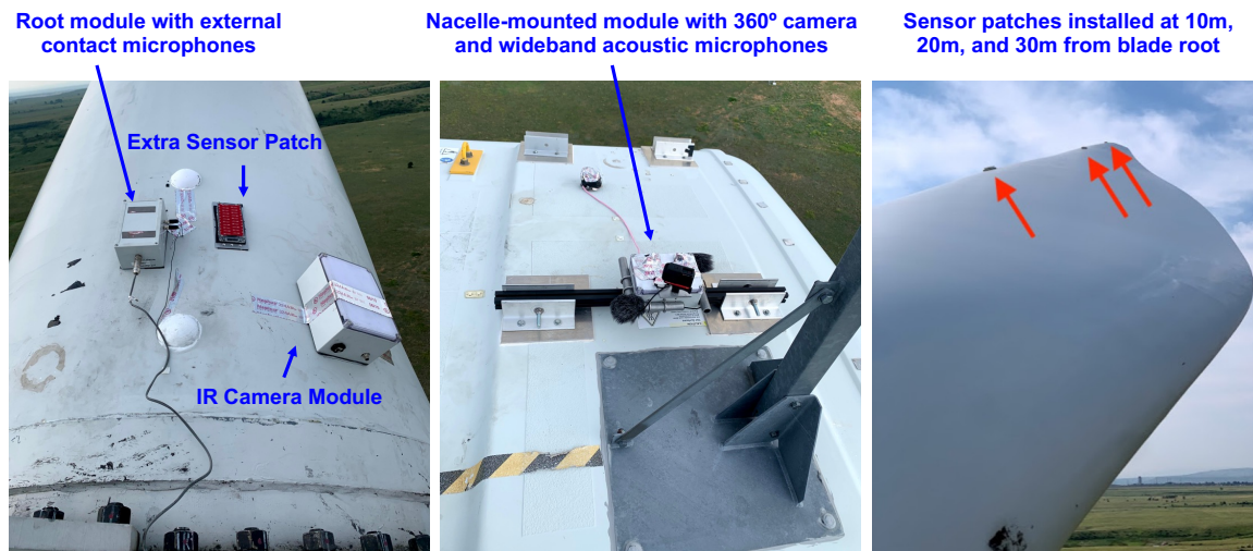
Figure 13. (left) Root module sensor, IR camera module, and extra sensor patch (for testing) installed near the root of a blade on a 1.5MW GE wind turbine; root modules installed on all 3 blades. (middle) A/V recording module installed on the top of the nacelle. (right) Distributed wireless sensor patches installed along the blade length.
